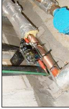
[Installation of the Vulcan completed]
