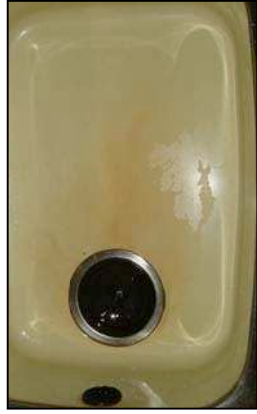
[Sink in the kitchen]
