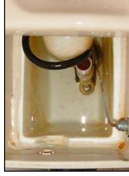
[Cleaned with sponge thirty minutes after the installation of the Vulcan]
