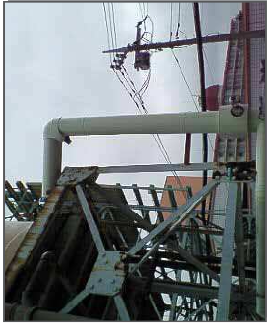
[Before installation of the Vulcan]
