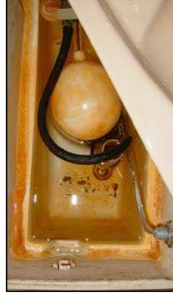
[Before installation of the Vulcan]
