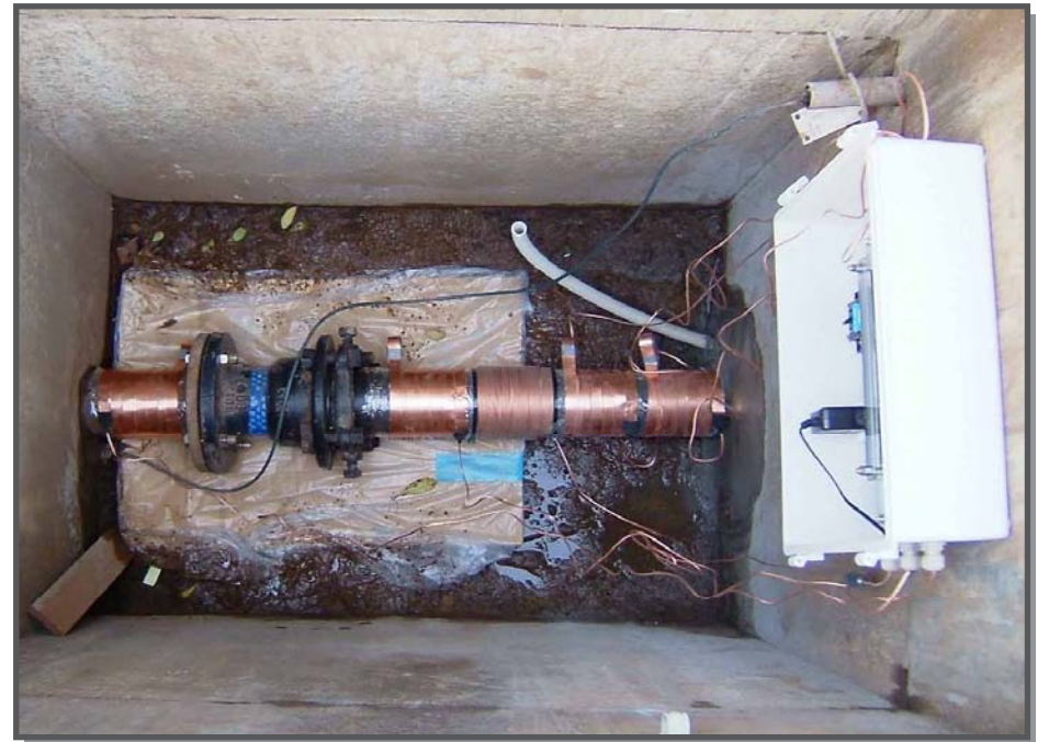
[Cable winding completed]
