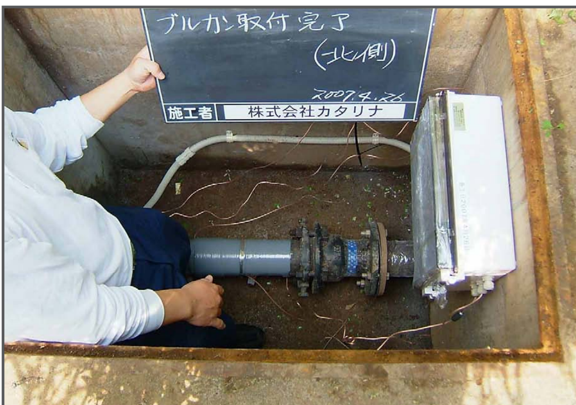
[Installation of the Vulcan completed]
